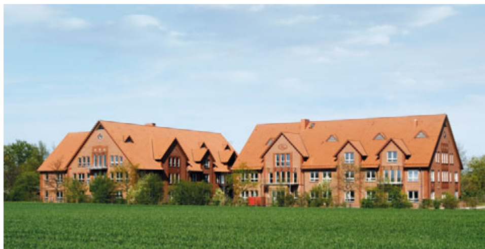
The "Laserhof" was originally built in 2002 with 1000 m 2 cleanroom production (building on the left side). After just twelve years in 2014 it became necessary to expand to 7900 m 2 in order to meet the growing demand for high power optics.
